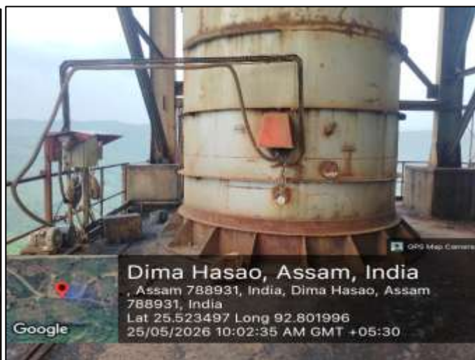
OCEMS at Coal mill stack
