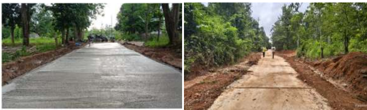
Cement Concrete Road construction
